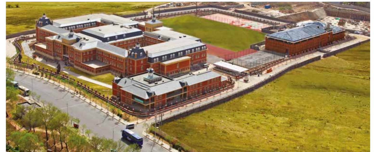
Wellington College, Tianjin, under construction
